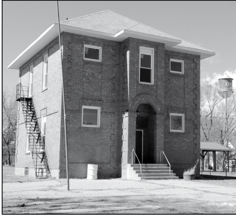
The Utica Town Board holds meetings in the former Utica School Building, which has been repurposed as the Utica Multi-Use Facility.
